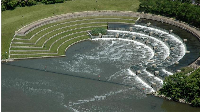
Figura 97. Infraestructura de reaireación y enfriamiento de agua: Sidestream Elevated Pool Aeration station in the Chicagoland Cal-Sag Channel and Calumet River (fte: Metropolitan Water Reclamation District).
